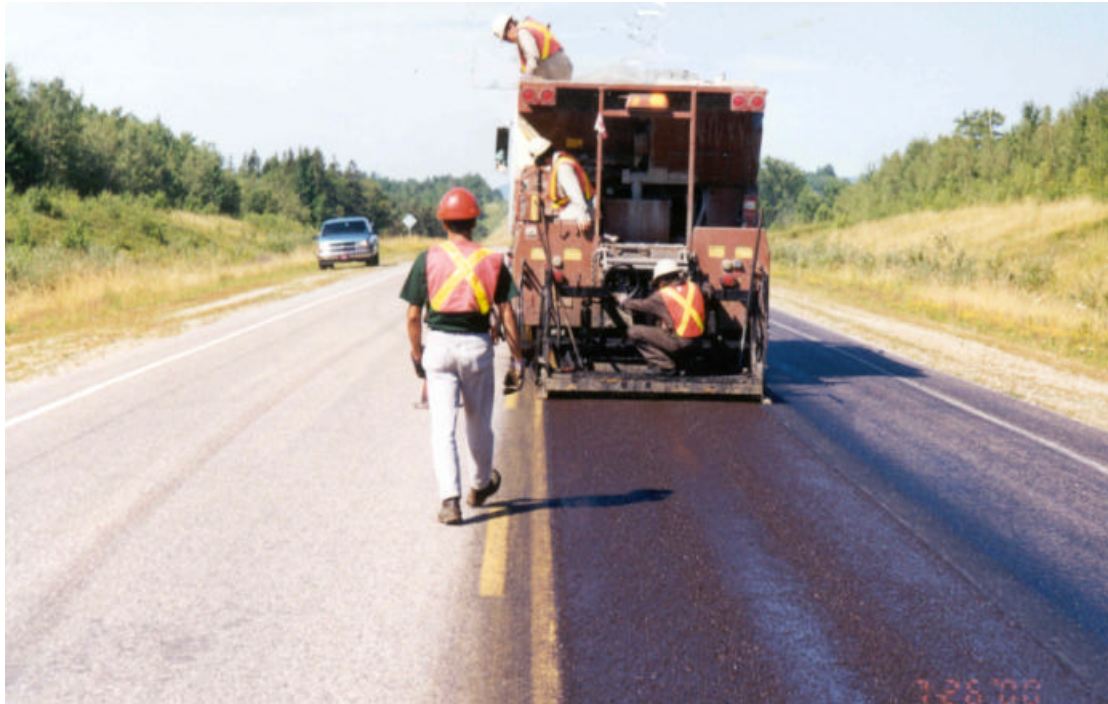
Figure 6. Rut Filling Operation
