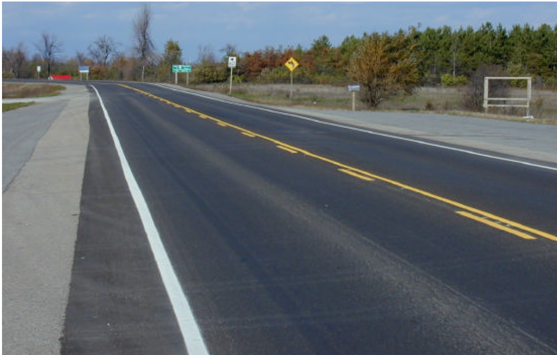
Figure 7. Micro-Surfacing after a few months of service
