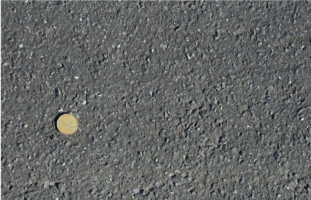
Figure 5. Micro-Surfacing Type II Surface Texture
