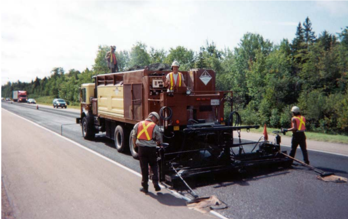
Figure 1. Truck Mounted Slurry Machine
