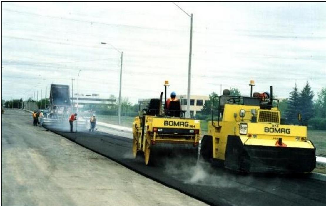
**PHOTOGRAPH 4: Compaction Equipment Rolling Hot Mat. Note Heating Vent and Skirts on Rubber Tired Roller to Aid in the Prevention of Pick-up.**
