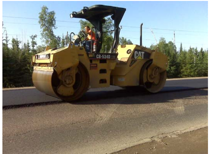
Mix Laydown – Compaction/Temperature
