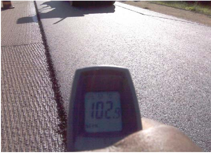
Mix Laydown – Compaction/Temperature
