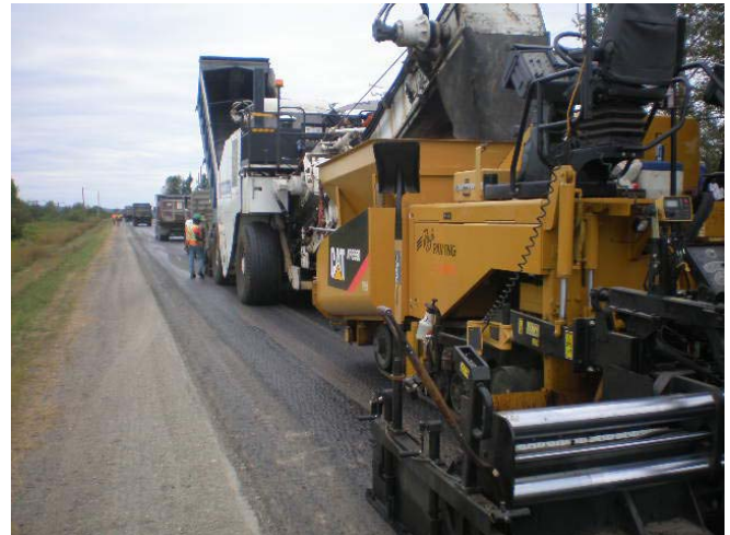
Pic 4: Shuttle buggy ensuring constant paver movement and smoother mat
