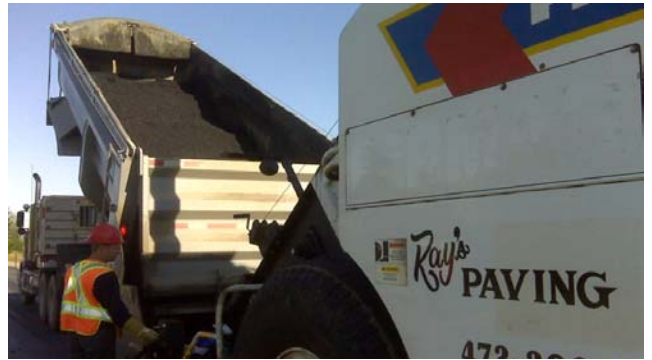
Mix Production – Discharge/Hauling
