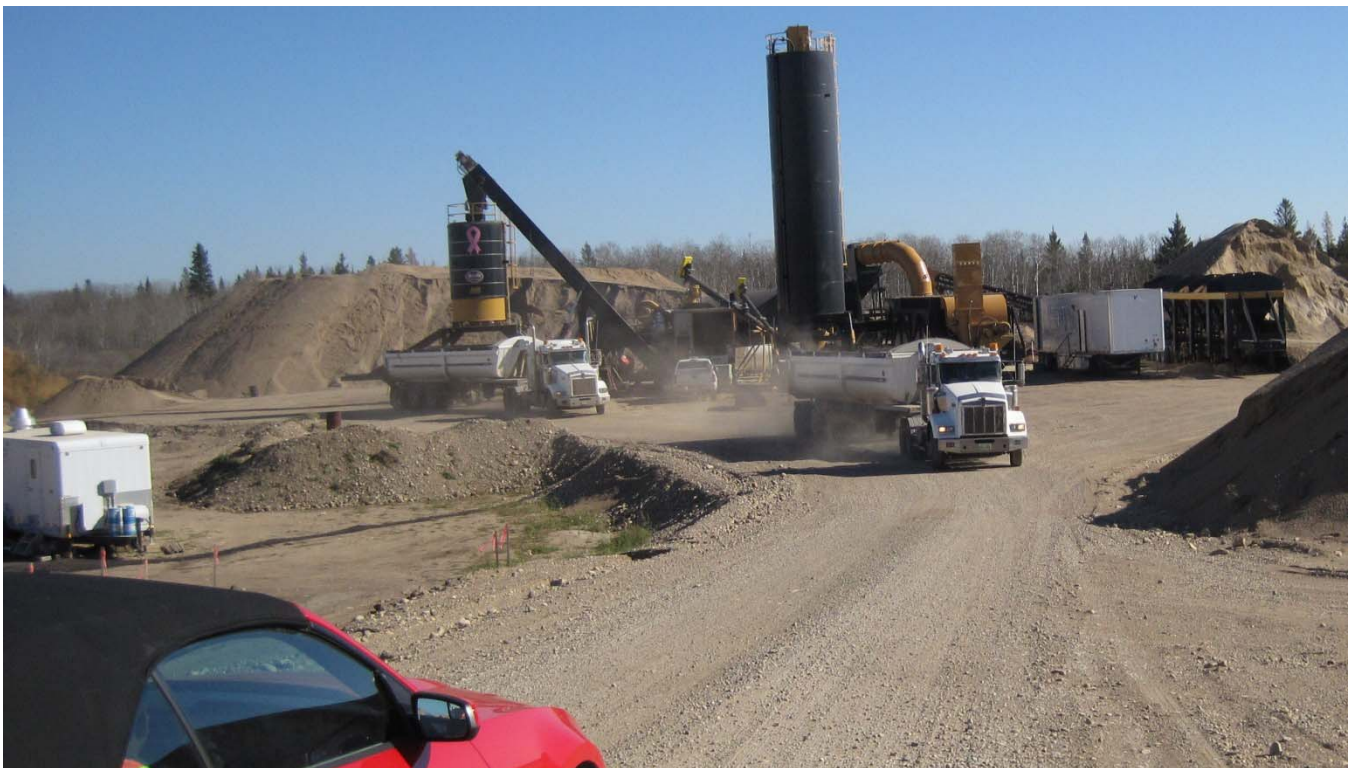
Morsky Plant (note the Saskatchewan Highways Lab trailer on the left)
