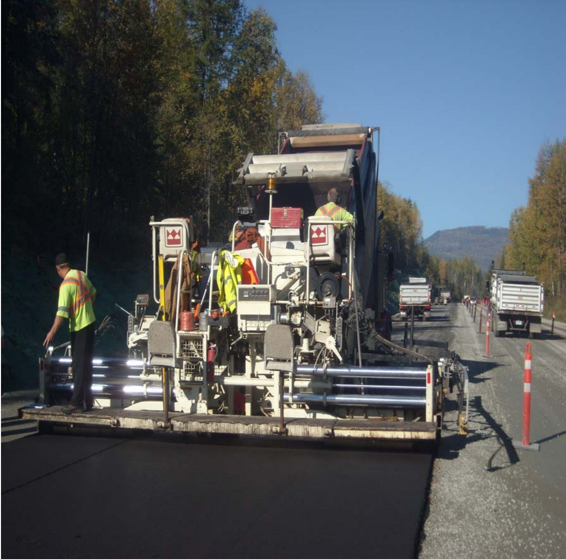
Selkirk Paving Crew, NO FUMES
