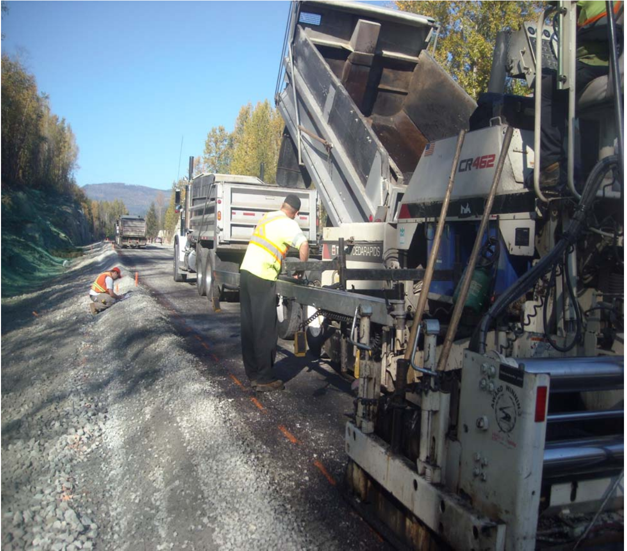
Selkirk Paving Crew, NO FUMES
