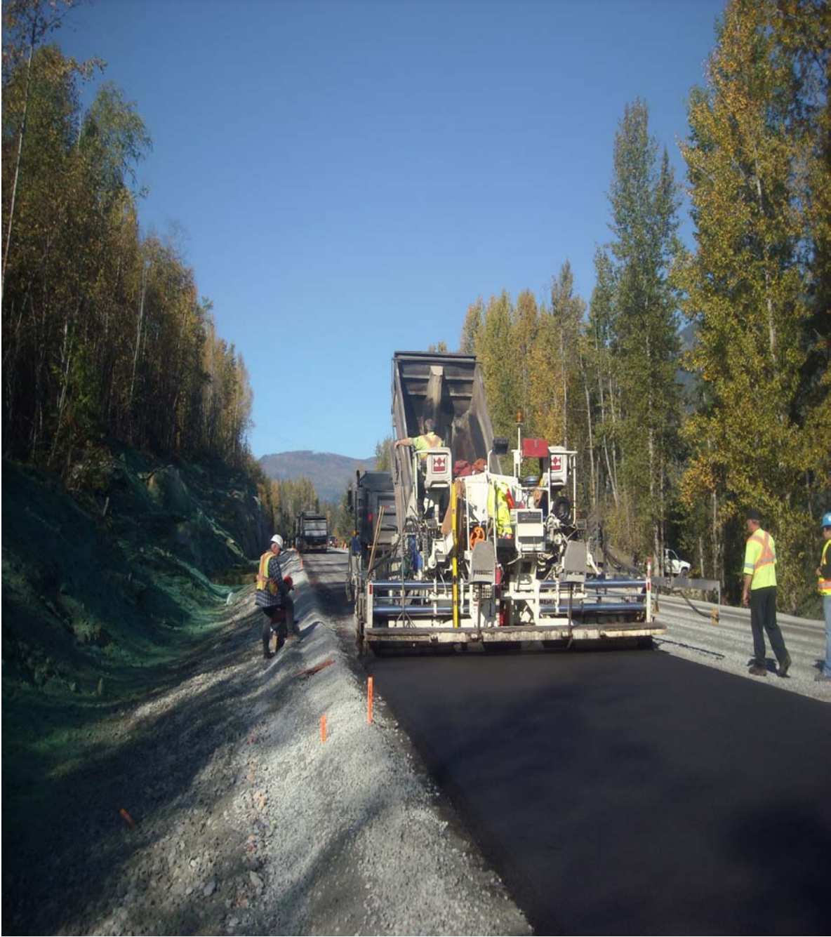
Selkirk Paving Crew No Fumes
