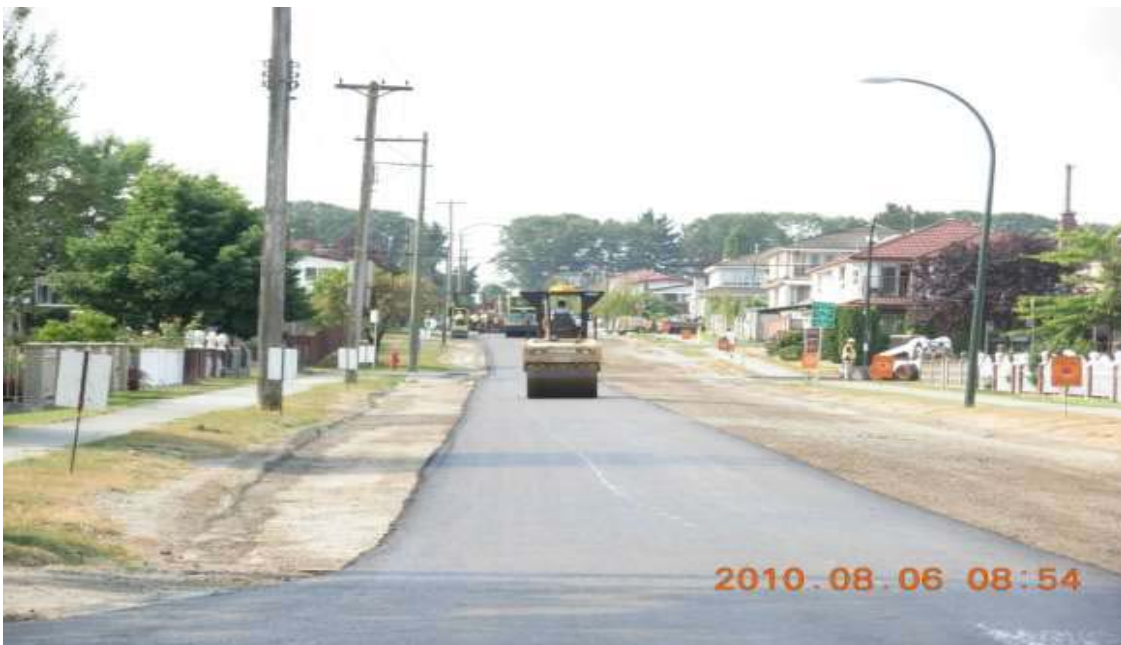
Fig 5: Final Compaction
