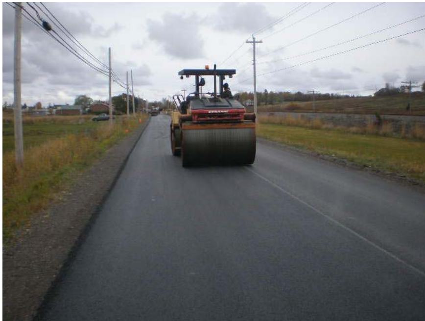
Pic 3: Nice uniform WMA mat on Trunk 2
