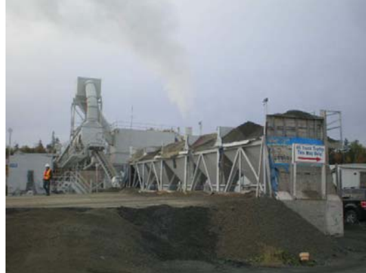
Pic 2: Cold feed bins had good bin-dividers to prevent x-contamination! Excellent!
